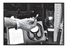
Check the gas pressure at the secondary regulator to make sure there's enough pressure for proper generator operation.
